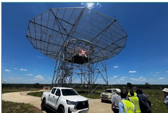
Instrument Landing System
