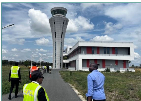
New Air Traffic Control Building
