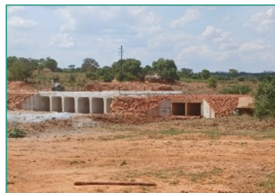
New culvert on Section 3 under construction in November 2023
