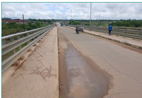
Narrow bridge deck with cracked surfacing and ponding of water (left), view eastwards showing new residential areas since construction of bridge (right)
