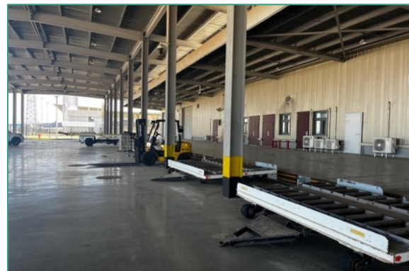
Air cargo facility
