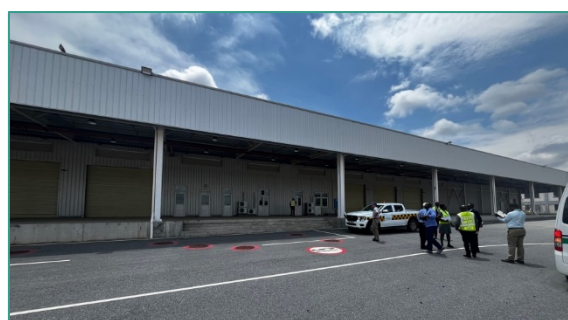
New cargo facility
