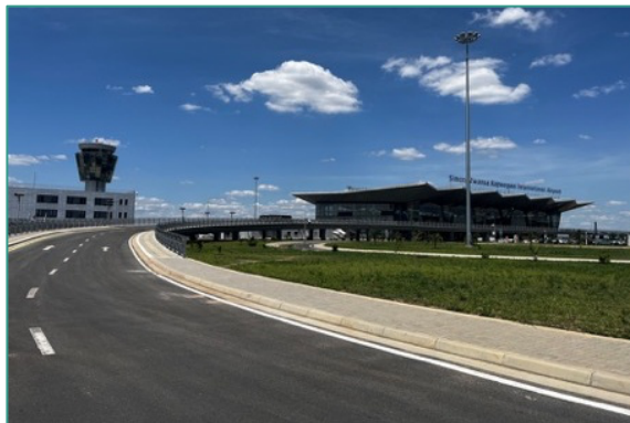
Vehicle access ramp
